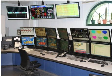
As part of the overall design, UConn also chose to place all of the PC’s in a remote cabinet outside the control room. This allowed for easier maintenance of the equipment and better thermal management.
